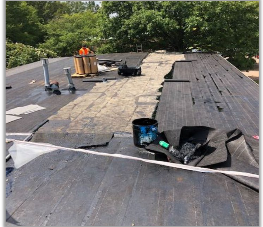
Roof renovation for Adult Education Building at Lawson State Community College
